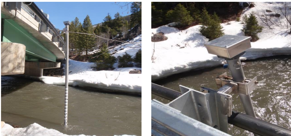
Figure 7. Bridge below Flat Rock Campground sonde housing ("boom")
