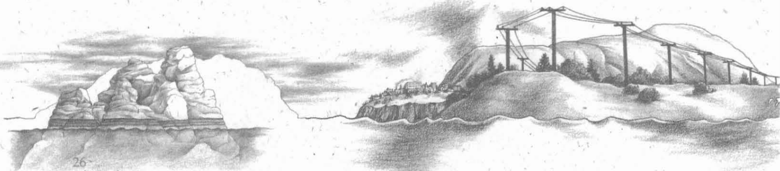
1937 "The transmission of electricity is making such scientific strides today that we can well visualize a date...when every community in this great area will be wholly electrified." —President Franklin Roosevelt dedicating Bonneville Dam.
