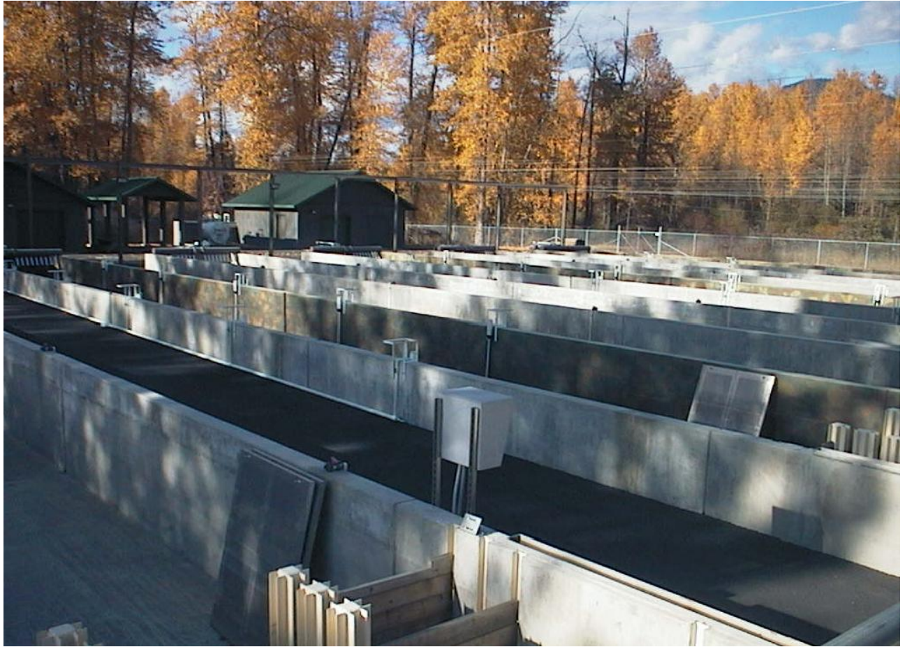
Figure F-4. Constructed Concrete Raceways - Easton Spring Chinook Acclimation Pond, YKFP
