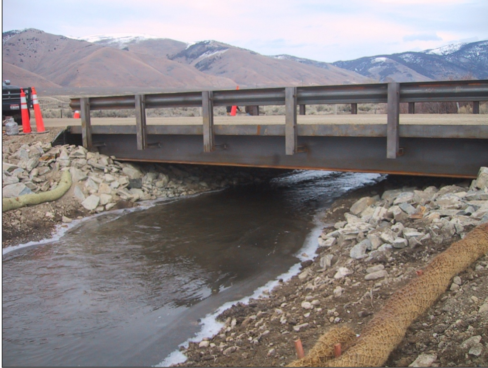
Figure 37. Canyon Creek Crossing After the Project.
